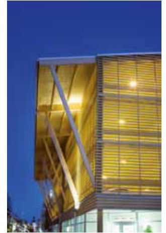
Martinsons supplied the frames for Sweden's first parking garage made of glulam timber, located in the timber town of Skellefteå, Sweden.
